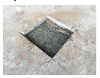
After removing concrete, auger or manually dig a minimum 24in/600mm diameter x 71in/1800mm deep hole.
