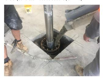
Fill the remainder of the hole with concrete. Ensuring that the application of concrete does not move the reo cage out of position.
