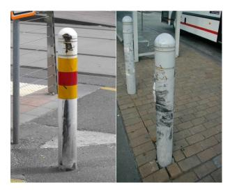
Check that the bollard is still vertical, if the bollard is not vertical the footing may have rotated in the ground or the bollard may have been bent by an over capacity impact such as a truck. The bollard may need to be removed from the footing to assess if the pipe is still straight.
