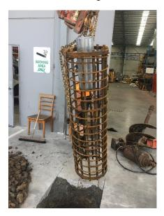
Insert the Omni-Stop Super Duty Security Bollard reinforcement cage, ensuring that the cage is at equal distance from the edges of the hole. Also ensure the top of the sleeve is level with the finished concrete surface.
