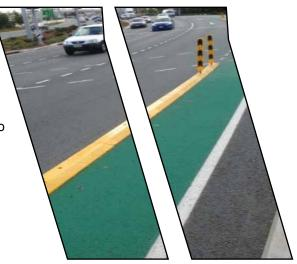
Cinar Kunduz, Project Manager at RoadTek, is very happy with the Saferoads separation kerb solution that directs vehicles to turn correctly and not cut corners and keeps vehicles away from a designated bike lane on a high traffic volume sweeping bend.
