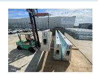
Barriers are only to be moved as a single item lift. It is recommended that barrier are moved with the use of a jib and chain and lifted at the centre lifting point of the HV2 Barrier.
