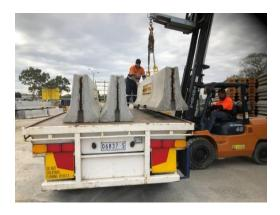
10.9 Ensure that the barriers are neatly positioned. This will ensure that the load is central.
