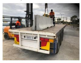
10.6 The next barrier is moved to the trailer and is placed on the left hand side of the centre barrier
