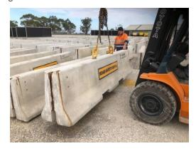
10.4 Using a spotter will assist in steadying the barrier and assist in a smooth transportation of the barrier to the vehicle
