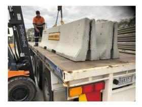
10.7 During the loading process of the T-Lok barriers, it is important to have a staff member on the deck of the trailer.
