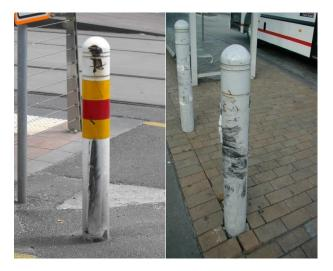
Check that the bollard is still vertical, if the bollard is not vertical the footing may have rotated in the ground or the bollard may have been bent by an over capacity impact such as a truck. The bollard may need to be removed from the footing to assess if the pipe is still straight. A closer visual inspection of the footing will be required to identify any cracking or breakage. Broken pavers are a tell-tale sign of footing damage.
