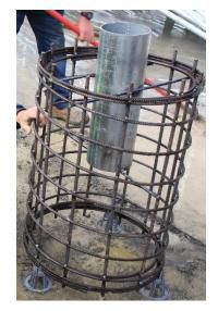
Insert the Omni-Stop Ultra Security Bollard reinforcement cage, ensuring that the cage is at equal distance from the edges of the hole. Also ensure the top of the sleeve is level with the finished concrete surface.
