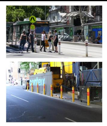
The Omni Stop Ultra Security Bollard can be fitted with a lifting ring to enable the bollards to be lifted out of the footing when used in a work zone. An Omni Stop footing cap is placed into the sleeve to allow for vehicles and pedestrians to traverse safely.
