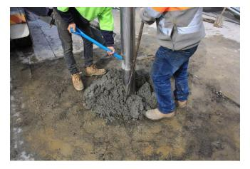
The concrete should be vibrated with a pencil vibrator to settle the concrete and remove air pockets.
