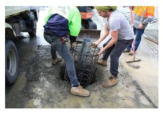
Use a spirit level to ensure that the reinforcement cage assembly is correctly positioned.
