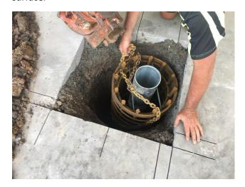
Use a spirit level to ensure that the reinforcement cage assembly is correctly positioned.
