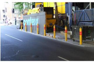
The Omni Stop Super Duty Security Bollard can be fitted with a lifting ring to enable the bollards to be lifted out of the footing when used in a work zone. An Omni Stop footing cap is placed into the sleeve to allow for vehicles and pedestrians to traverse safely.
