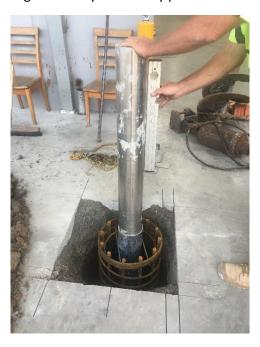
Note: using a 6in/150mm x 57in/1450mm light weight galvanised pipe placed into the cage to check that the bollards will be vertical may assist.
