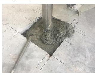
The concrete should be vibrated with a pencil vibrator to settle the concrete and remove air pockets.
