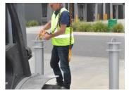
Once the bollard is on the ground, remove the lifting hooks
