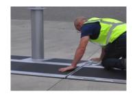
Allow the two bollards to join at the central connector points.
