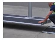
Working downstream of the first bollard unit, unload the second unit and align the connectors while lowering the unit into place.
