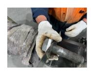
Place a washer onto the bolt and slip on the flange ring.
