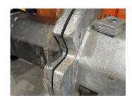
Ensure that the stub and the pole are at the correct orientation to allow fitment of hardware.
