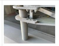
Attach a Galvanised M24 washer and M24 Nyloc nut, doing up finger tight. Repeat the process with the remaining bolts.
