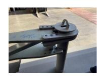
Using a galvanised M24 x 120 bolt and M24 washer place the bolt through the predrilled hole and ensure that the bolt passes though the top "U" plate, Gate Rail and bottom "U" plate. Repeat the process until all 6 bolts have been inserted. On occasion the bolts will not sit flush. Simply use the Air Impact Wrench with the 41mm socket and the bolts will sit flush.
