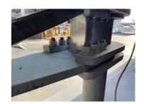
Using the M24 bolts, washers and nylocs (as per the top plate), insert the bolts in the inverted position and do up finger tight.
