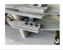
Place the bottom "U" plate into position. The "U" plate will remain in position on an angle as it will grab against the shaft of the bollard.
