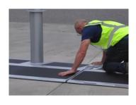
Allow the two bollards to join at the central connector points.
