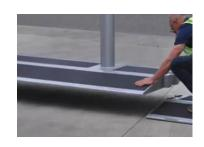
Place the bollard in the correct position. During this stage all operators are to remain clear of the lift.
