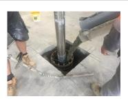
Pour concrete into the space surrounding the reo cage to approx. 12in / 300mm and then re-check levels. (Concrete must be 5000PSI / 32MPa).
