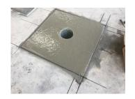
Finish off by screeding the concrete surface and if applicable replace pavers around installed bollard.
