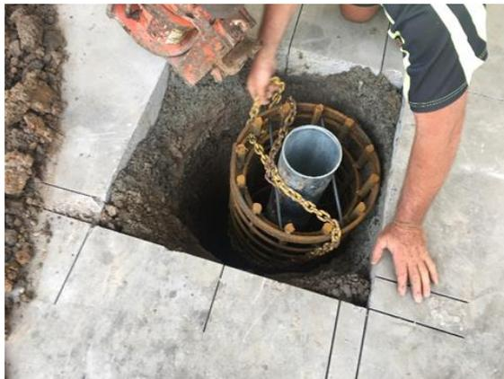
Use a spirit level to ensure that the reinforcement cage assembly is correctly positioned.
