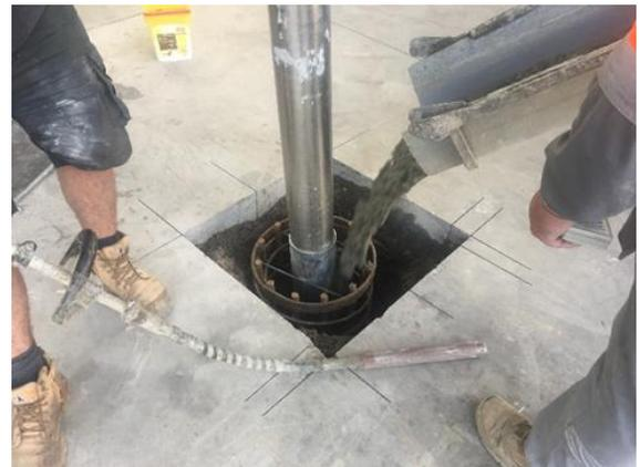
Fill the remainder of the hole with concrete. Ensuring that the application of concrete does not move the reo cage out of position.
