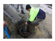
Pour concrete into the space surrounding the reo cage to approx. 12in / 300mm and then re-check levels.
