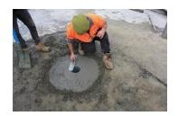
Finish off by screeding the concrete surface and if applicable replace pavers around installed bollard.
