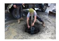
Place 4 reinforcement spacers under the cage to allow the reinforcement cage to sit clear of the sub-soil. Insert the Omni-Stop Ultra Security Bollard reinforcement cage, ensuring that the cage is at equal distance from the edges of the hole.
