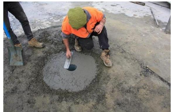
Note: If paving is to be placed over the top of the footing, the excavation must be deep enough to ensure that the concrete footing is minimum 40in/1000mm deep and 28in/700mm diameter.
