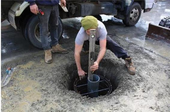
Note: using a 6in / 150mm x 57in / 1450mm lightweight galvanised pipe placed into the cage to check that the bollards will be vertical may assist.
