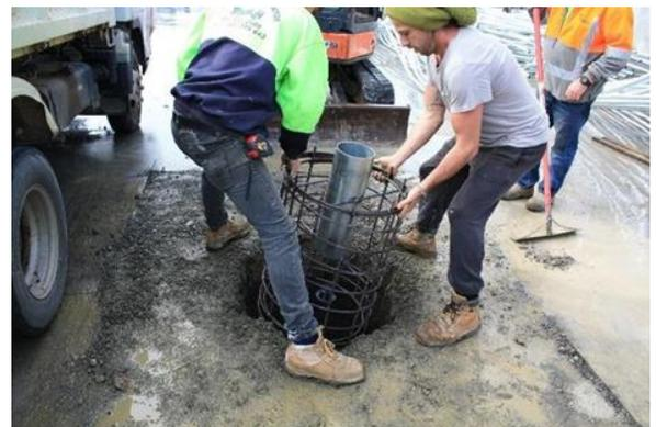
Use a spirit level to ensure that the reinforcement cage assembly is correctly positioned
