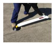
Place the base and butyl pad over the holes and insert the 150mm Coach bolt with flat washer. Using the Ratchet and Socket screw down until firm against the base;.
