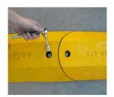
Place adjoining segment of kerb on to the other leg of the U-bolt
