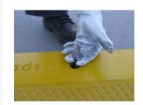
Using epoxy and caulking gun, insert nozzle into each hole and insert epoxy. Saferoads recommends 3 caulks per hole.
