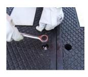
Finish tightening coach bolts using a ratchet socket wrench with a 17mm socket. Note: ensure this step is completed not too long after the previous step as the epoxy will set.
