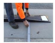
Place steel fixing angles into position with corner sections slotted into place
