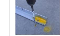
Insert orange nylon plug (ramset ultralong) into hole. Slide angle bracket back over hole and insert ultra-long screw Remove all rubber segments from one side and swivel angle bracket to one side to expose painted locations for fasteners. Repeat drilling and cleaning
