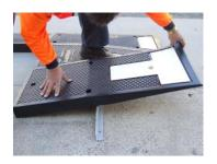
Place steel fixing angles into position with centre sections slotted into place
