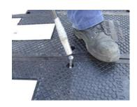
Quickly re-instate the segment into the correct position, lining up the fastener holes.
