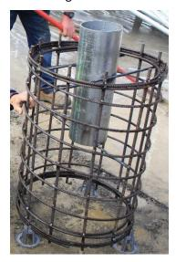
Insert the Omni-Stop Ultra Security Bollard reinforcement cage, ensuring that the cage is at equal distance from the edges of the hole. Also ensure the top of the sleeve is level with the finished concrete surface.
