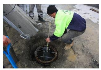
Fill the remainder of the hole with concrete. Ensuring that the application of concrete does not move the reo cage out of position.
