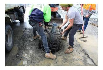
Use a spirit level to ensure that the reinforcement cage assembly is correctly positioned.
