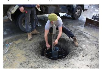
Note: using a 6in/150mm x 57in/1450mm light weight galvanised pipe placed into the cage to check that the bollards will be vertical may assist.
