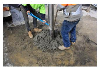
The concrete should be vibrated with a pencil vibrator to settle the concrete and remove air pockets.
